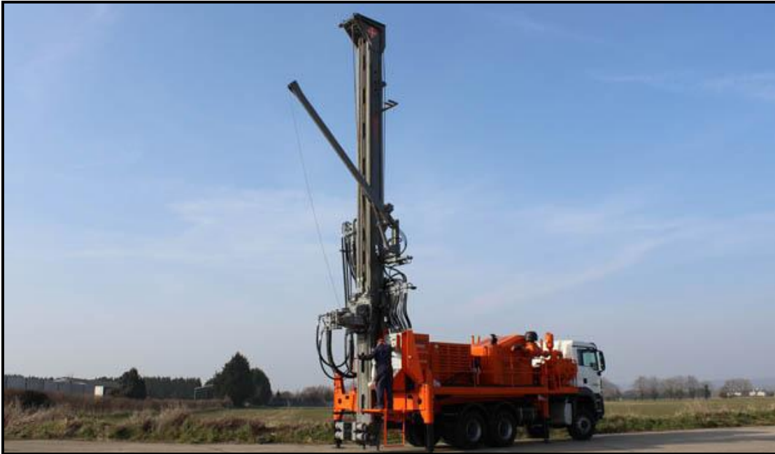
Figure 4 - Photograph of rig vehicle.
